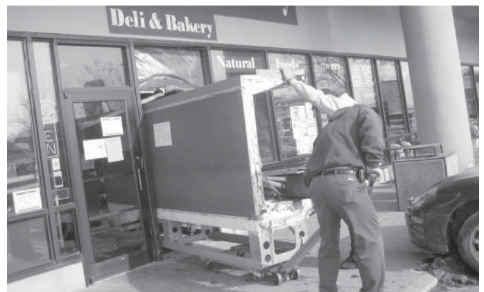
A-1 Refrigeration crew carefully removes retired coolers.
